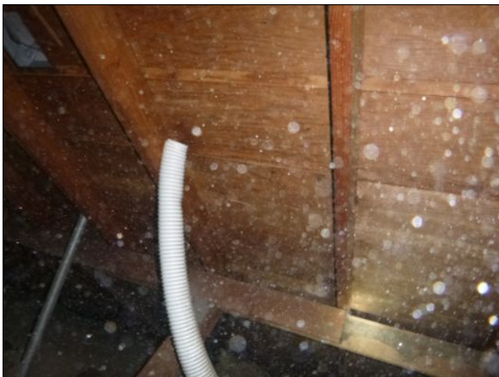
Exhaust duct terminates in attic. Hallway bathroom
