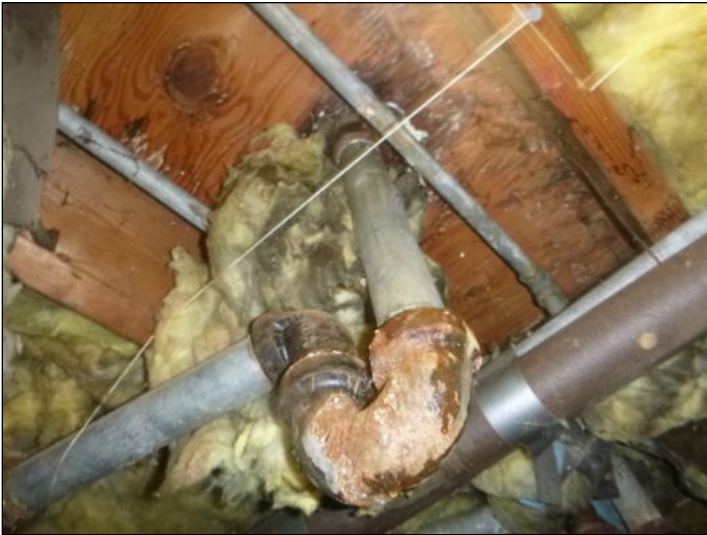
Leak in Drain lines or shower pan. Located under master shower.
