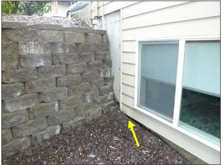
Clearance between the ground and the siding is inadequate.
