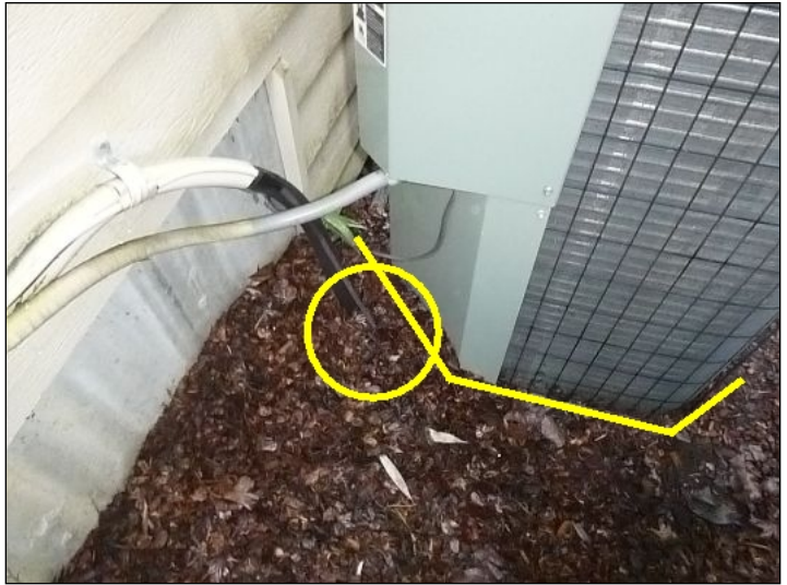
Remove bark around heat pump
