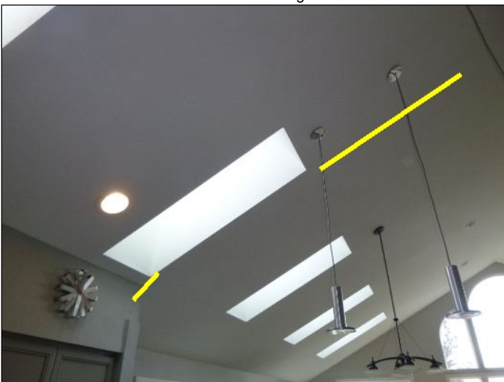
Cracks in ceiling.
