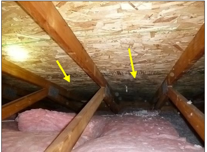
Roof sheathing is stained.
