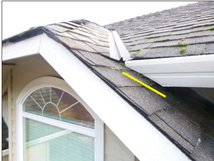
Gutter drains directly onto the shingles.
