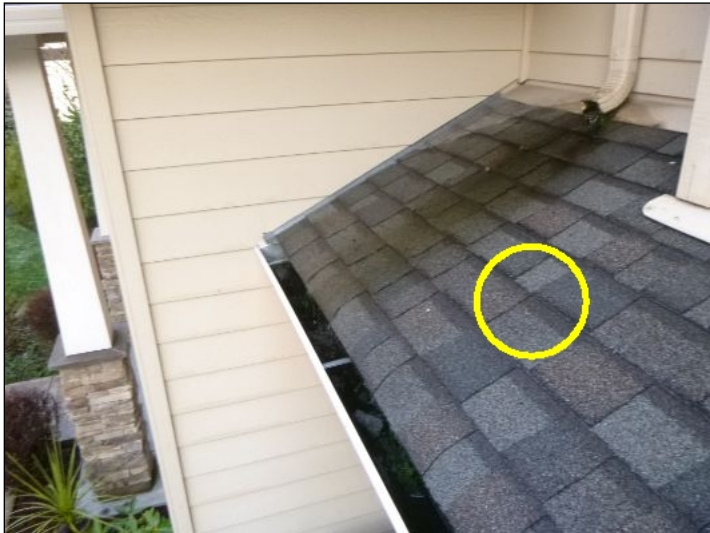
Nail sticking out of the shingles.
