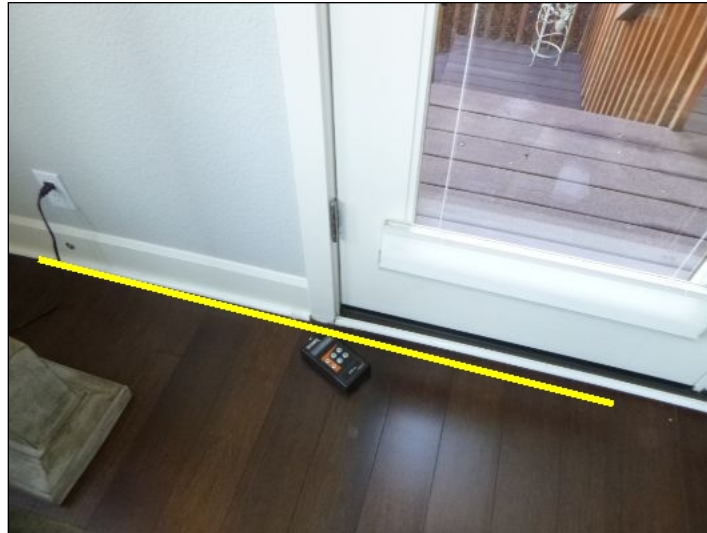
Moisture levels in the floor are elevated.
