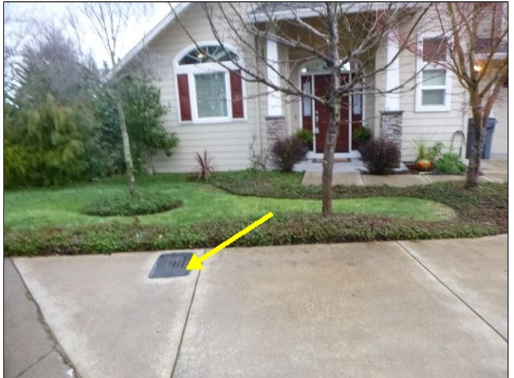
Main water shut-off location.
