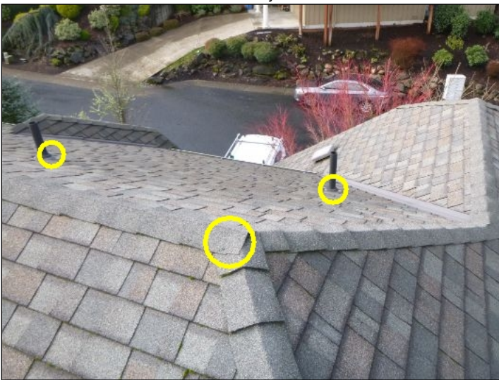
Fasteners are not sealed.
