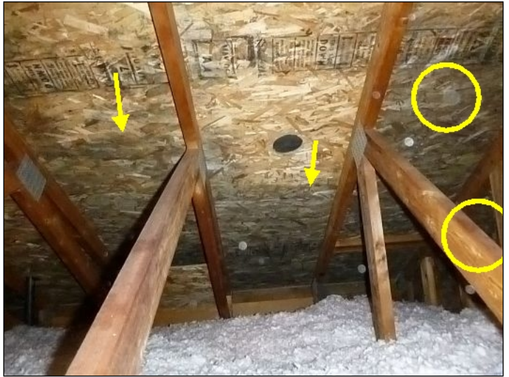
Roof sheathing is stained.
