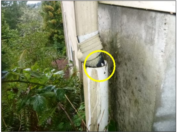
Reconnect downspouts at underground drainage system.
