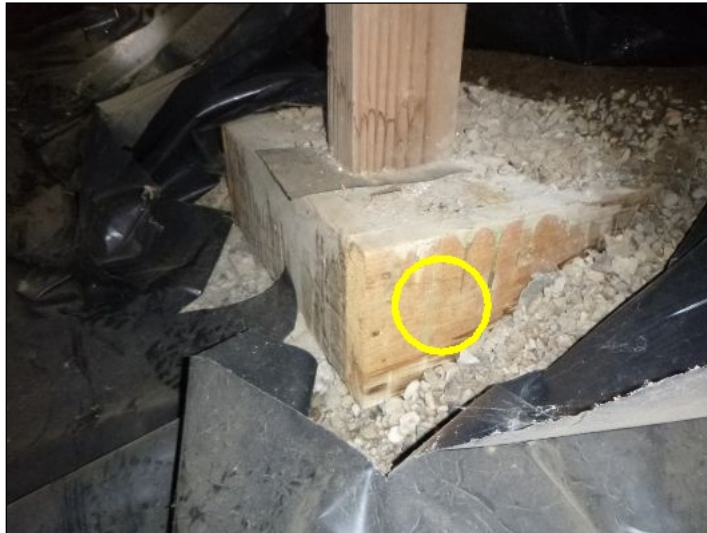
Wood debris in crawlspace.
