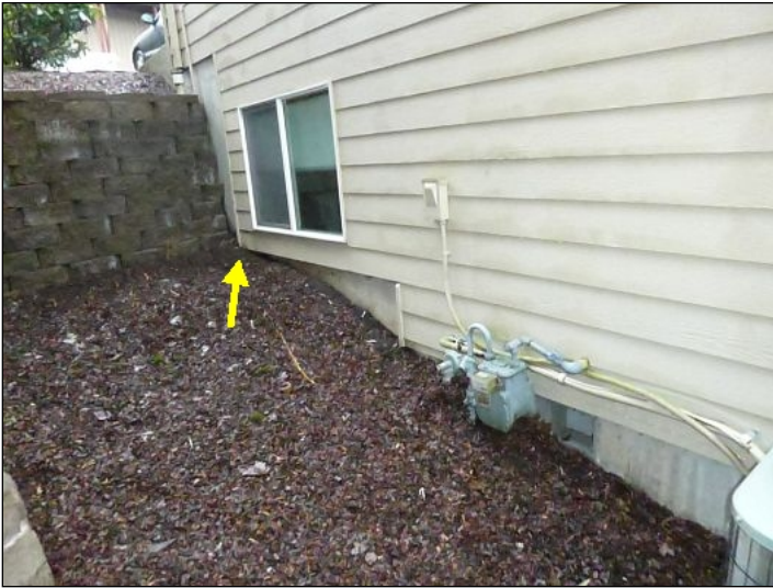
Main gas shut-off location.
