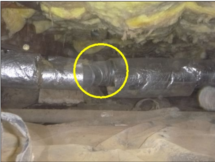
Duct insulation is damaged.
