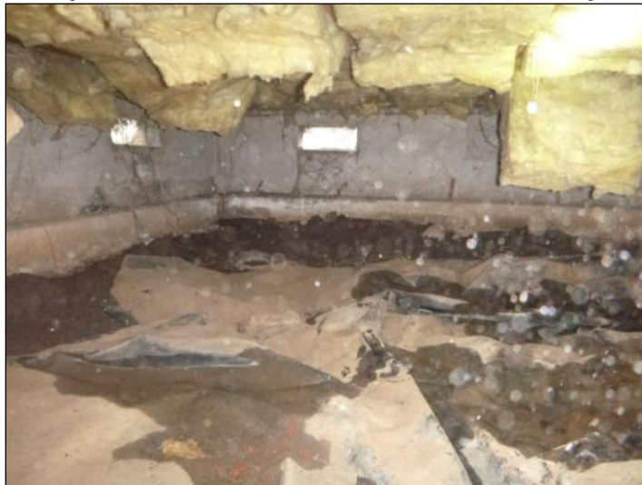
Pooling water in crawlspace. Displaced vapor barrier.
