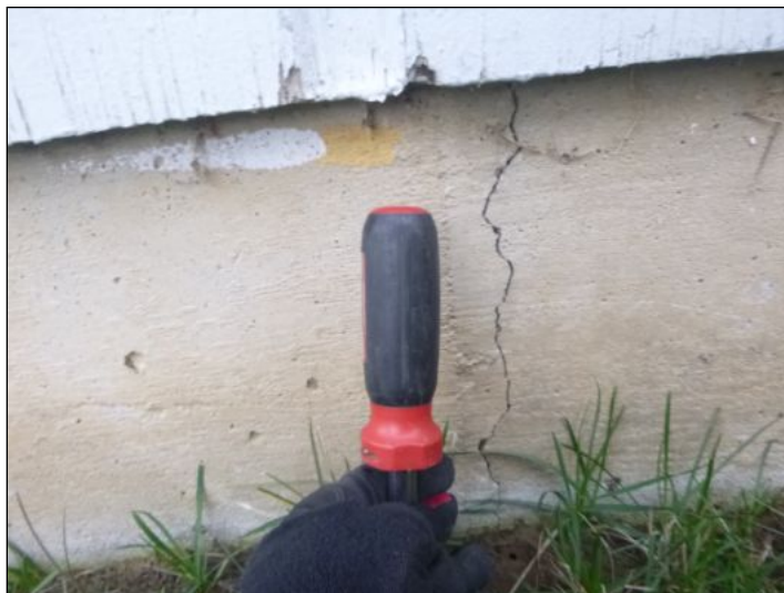
Cracks in foundation.
