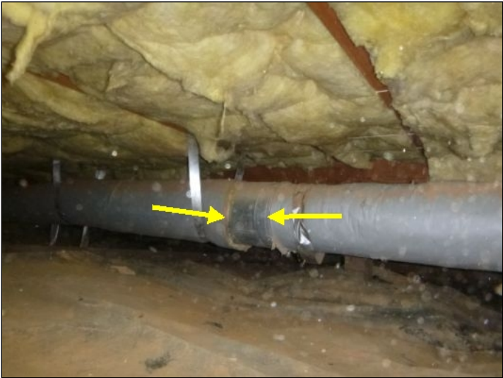
Duct insulation is damaged.
