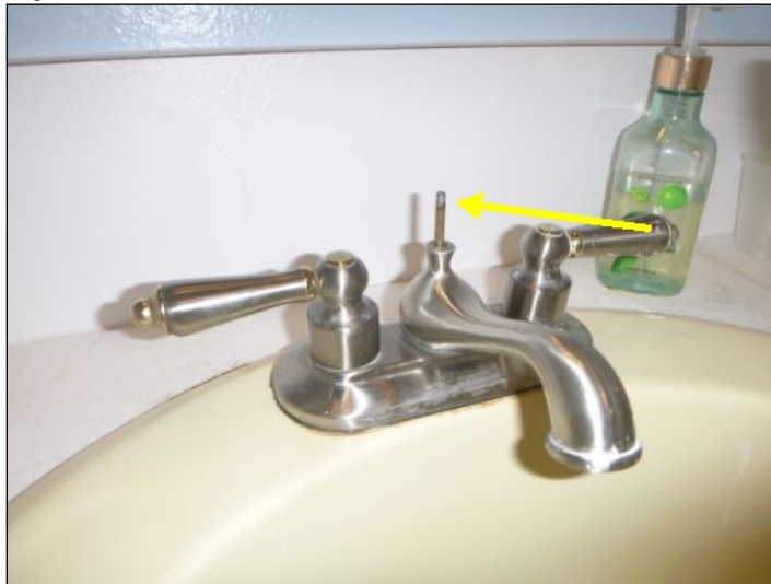
Stopper is missing knob.
