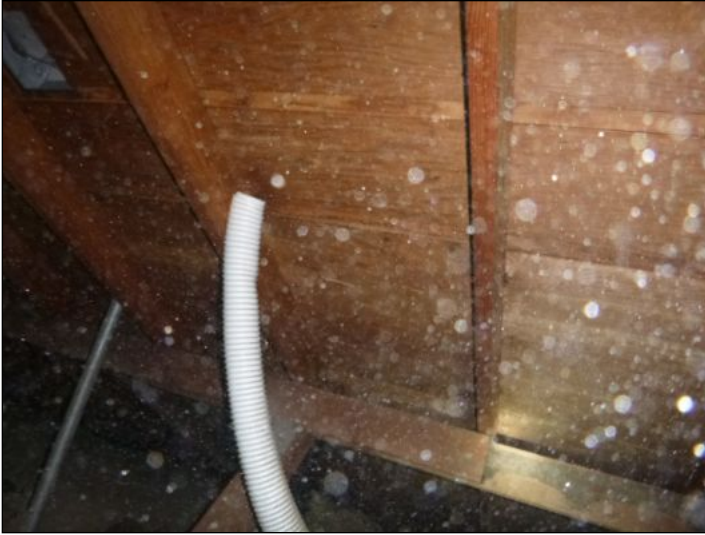
Exhaust duct terminates in attic. Hallway bathroom
