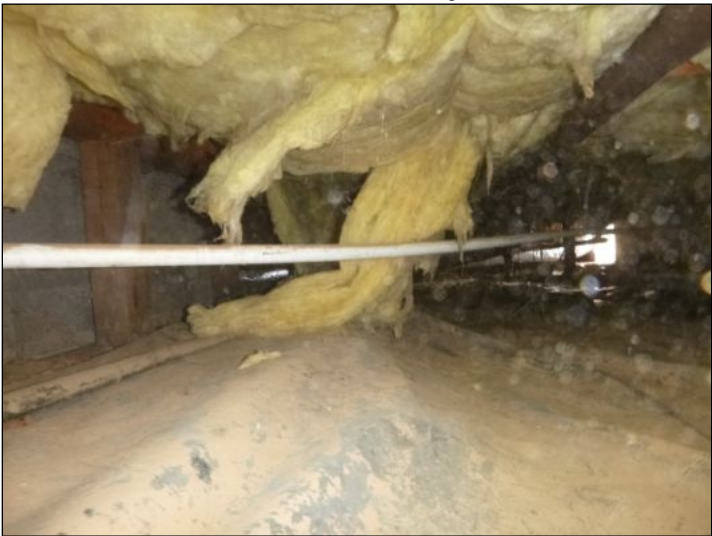
Missing or hanging insulation in a few areas..
