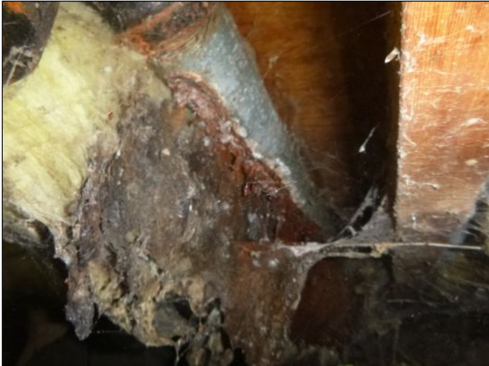
Leak in Drain lines. Under kitchen
