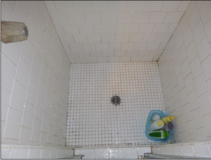
Grout is deteriorating. Loose tiles.
